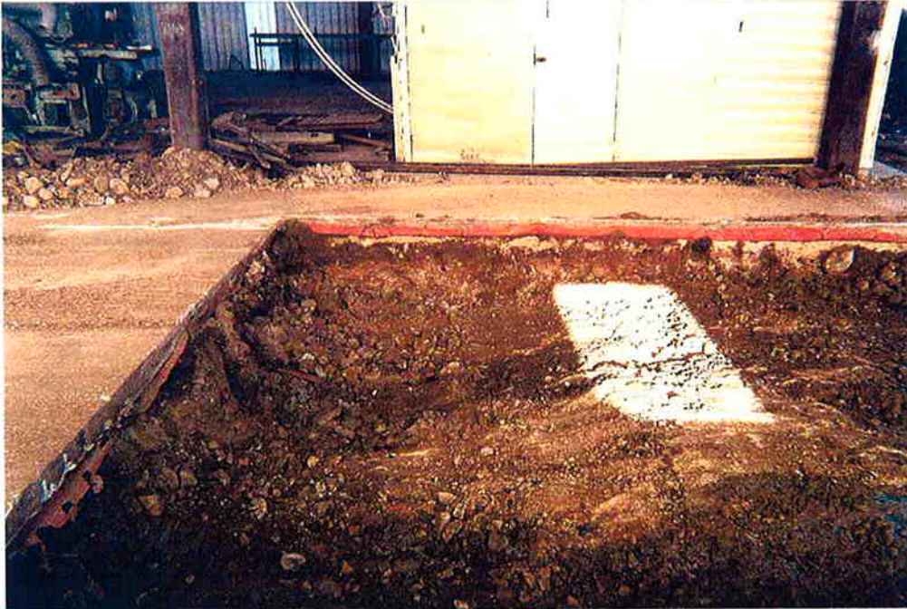
Plate 5: Looking to the north eastern corner of the excavation
