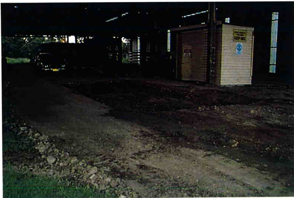
Plate 6: Looking north east across the excavation
