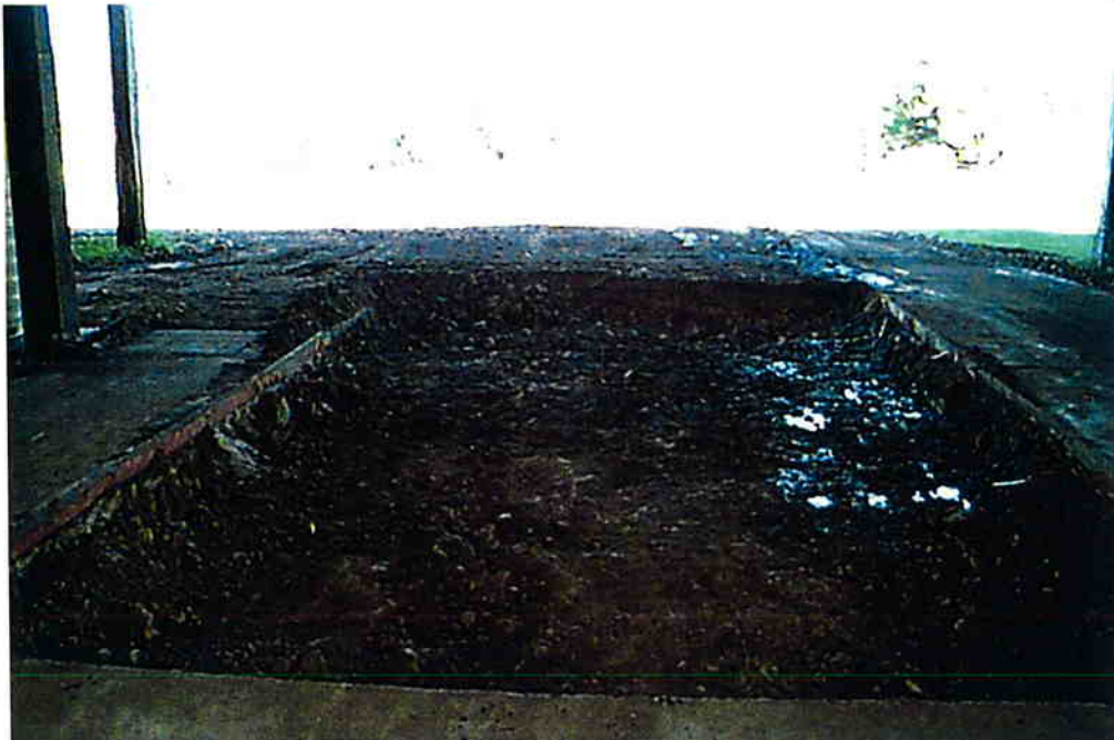
Plate 2: Looking south across the excavation.
