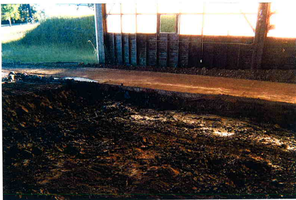
Plate 4: Looking to the south western corner of the excavation
